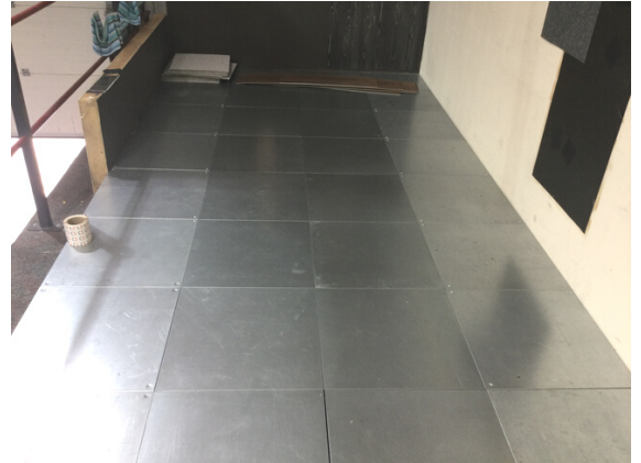
Raised metal access flooring after uplifting flooring installed using IOBAC Adhesive-Free MagTabs®
